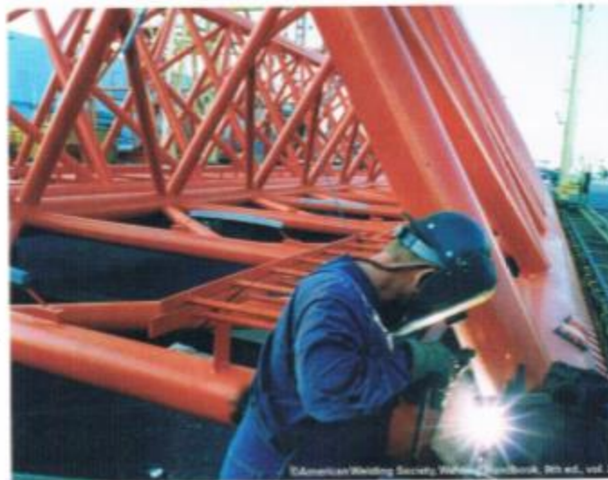
Shielded metal arc welding (or "stick welding")
