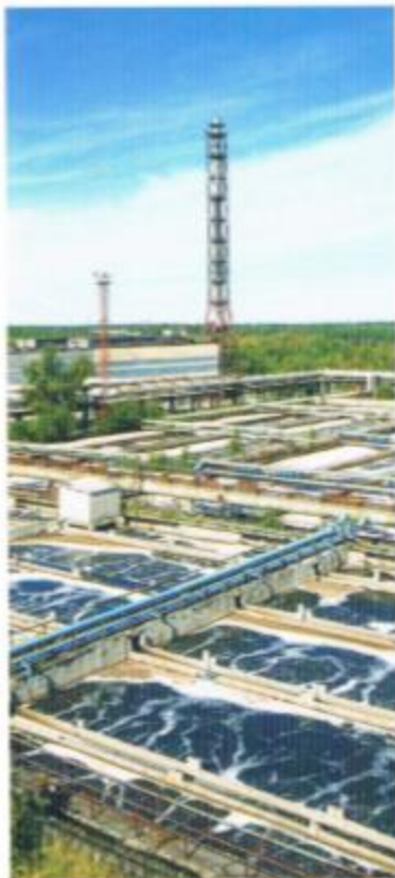
Water treatment facility
