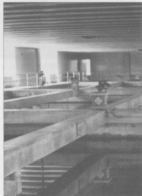
Right: Water is further cleaned in filter beds, where it percolates through a deep layer of sand.
