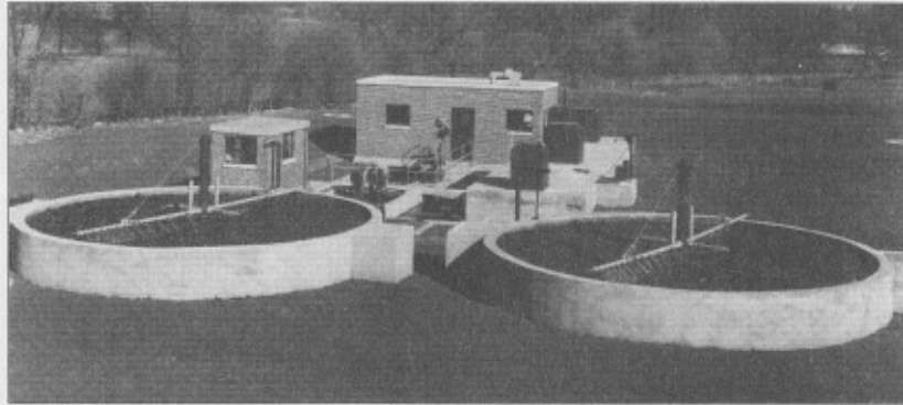
A small sewage treatment plant.
