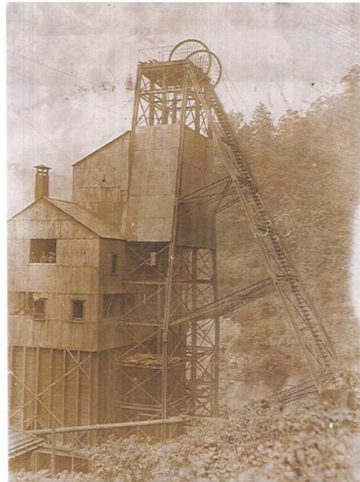
The smokeless coal formerly mined from the land of the BSA Summit fueled the steam shovels, steam drills, steam trains, and steamships that built the Panama Canal in 1904–1914. This photo shows a mine and tipple. Coal was lifted from the mine to the surface and prepared for shipping.
