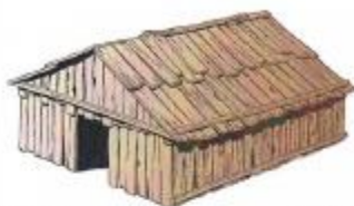
To build a plank house, the parts were grooved and fitted together to support one another.
