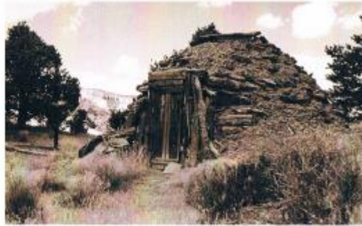
A Navajo hogan made of logs, small branches, brush, cedar bark, and earth
