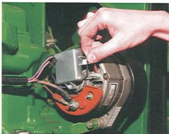
Inspect electrical wiring when the equipment is cold. Be sure connections are solid and no wires are abraded.
