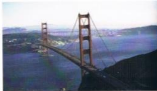
Golden Gate Bridge
