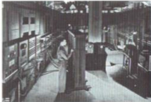
The U.S. military used first-generation digital computers like this ENIAC to calculate trajectories of artillery shells and to help build weapons.
