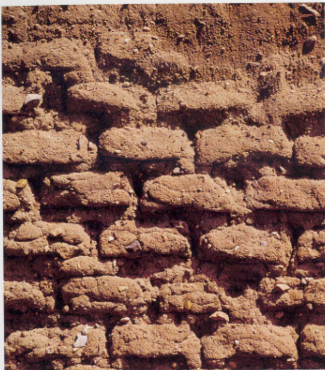
The adobe bricks used to build walls in some ancient civilizations were one of the first composite materials.
