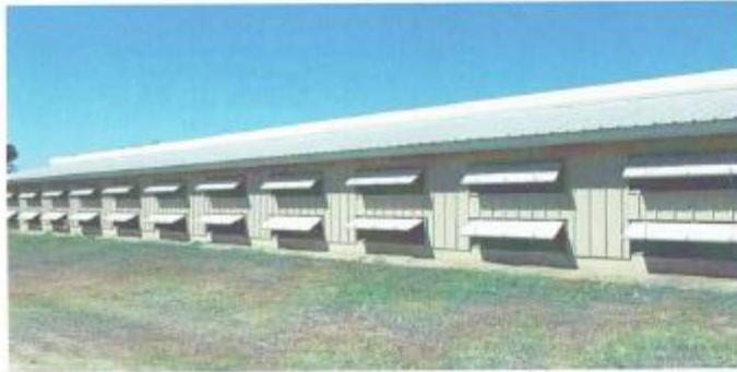
Layer and broiler houses protect birds from the elements. Most houses today, such as this layer house, are well-ventilated and well-insulated and have controlled temperature and automatic lights, feeders, and waterers.
